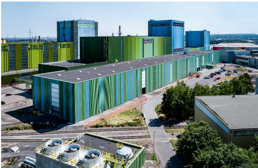
New hot dip coating line in Dortmund
